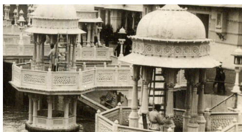
6796 C with workmen and ladders
