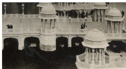
6796 C without workmen and no ladders
